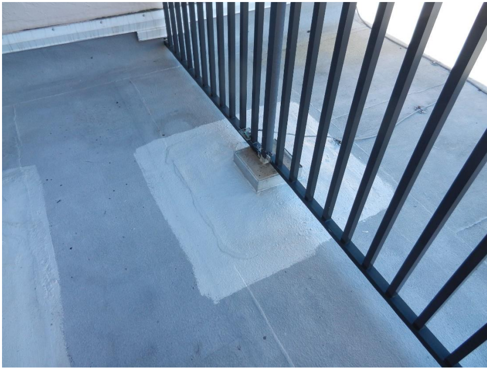
Areas of Maintenance
