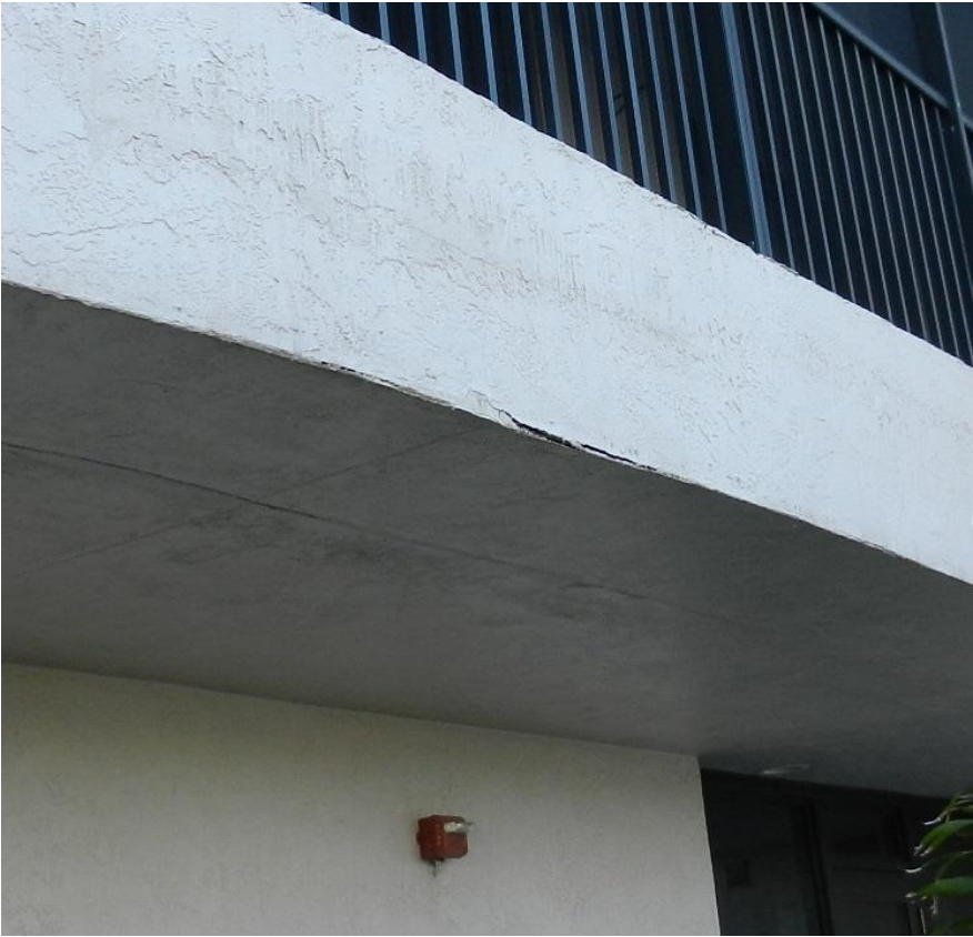
Rust Stains at the Northwest and Southwest First Floor Overhang
