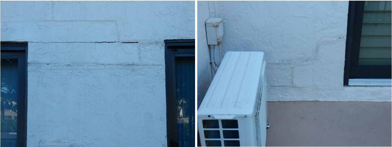
Continued Settlement at the Ground Floor Cabanas
